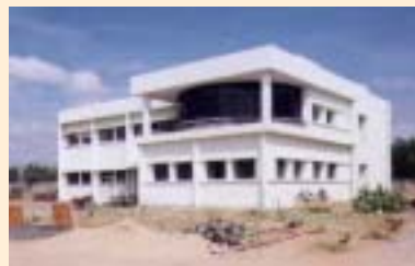
Nuclear Desalination Demonstration Plant (Capacity : 6300 cubic metre per day) set up at Kalpakkam, Tamil Nadu
