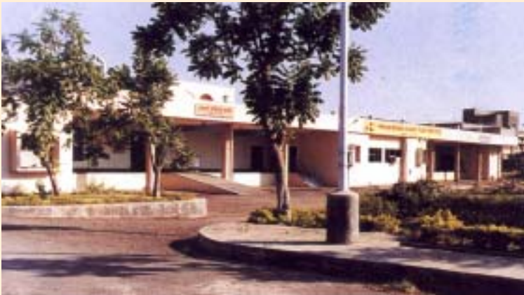
BRIT's Plant for radiation processing of spices at Navi Mumbai
